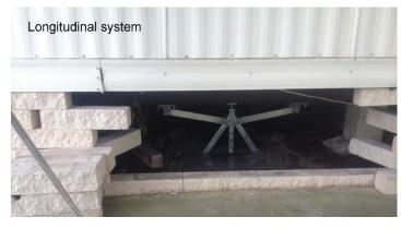
Lastly, we have longitudinal stabilizers. Often called X/I's, these are designed to resist horizontal winds against the end of your home. These must be connected to a clip that is welded to the I-beam.
