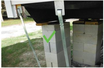
The second tie-down type of anchoring that may added is attached to a home's vertical tie connector, or overhead strap. Many homes are manufactured with these connection points built within the siding of the home. Where possible, installers will add straps to these points as well.
