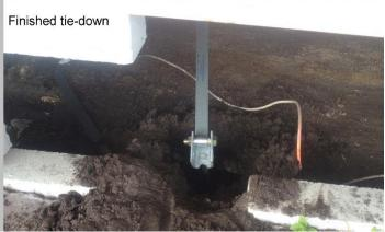
either a 4-foot or 5-foot long galvanized steel screw which is set into the ground, along with a stabilizing anchor plate. The strap is clamped to the I-Beam under your home and ratcheted to the anchor at a specific angle to reduce home movement.
